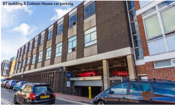
BT building & Colman House car parking
